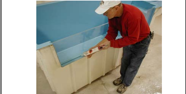
5. Use remaining caulk to fill in gaps on the inside and outside of window channel.
